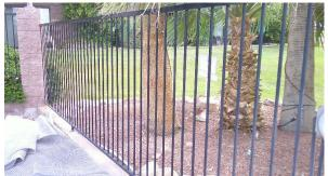
Budget to repair metal fencing. Noted approximately (5) sections/places where in need of repair due to spray irrigation, rusting.
