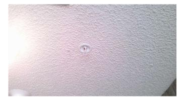
Sprinkler heads should be tested per NFPA 25. There are different types of sprinkler heads. When they should be tested depends on the type of head. Recommend Association consult with their fire protection vendor to determine if and when testing should be done.
