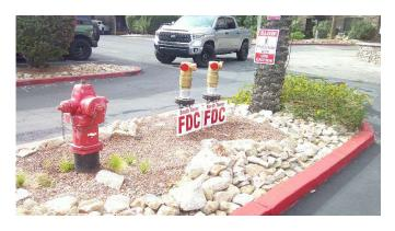
Budget to replace (2) 4" check valves & (2) 4x2 - 1/2" fire dept connections.
