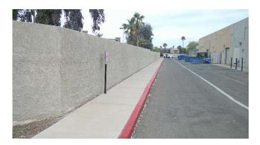
Poor condition. Budget to paint the perimeter stucco walls. Noted chipped, fades and in need of paint.
