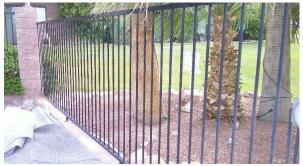
Poor condition. Budget to paint doors, metal stair railings, metal on balconies, and all other metal components on buildings and at pool.
