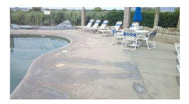
Poor condition. Budget to recoat pool deck. Noted faded and stained.
