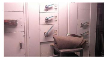
Working condition. Budget to replace (4) 400 amp breaker boxes in equipment rooms.
