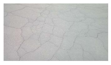
Budget to remove & replace asphalt. Extensive alligator cracking, however only a minor amount of break-up. If more areas begin to break-up, it is anticipated that the pavement will need to be removed and replaced. Future updates to this study should continue to evaluate the pavement and make appropriate adjustments in the useful life.
